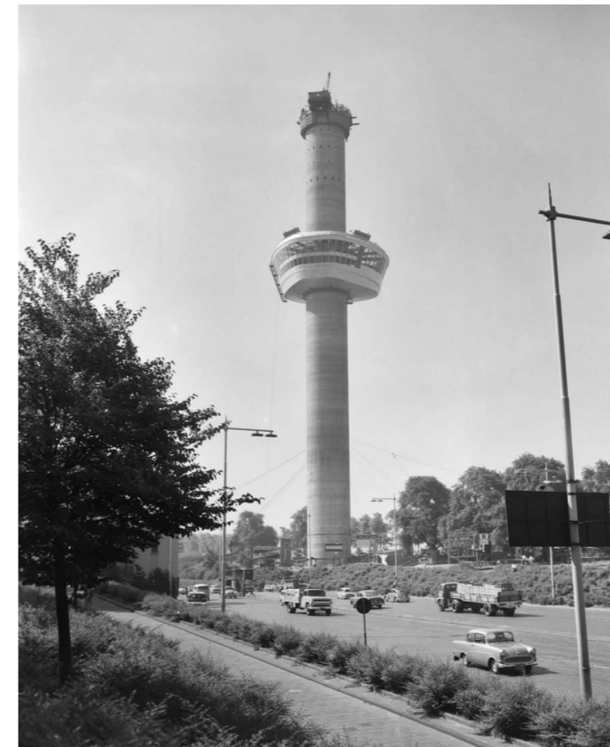
Figure 20. Construction of the Euromast, 1959. 18
