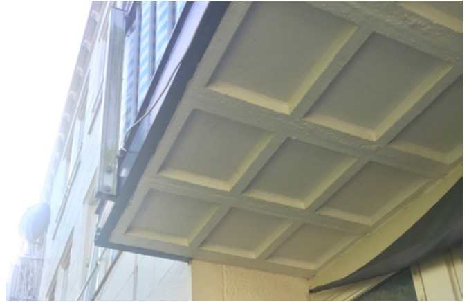
Amount : strip (A) 12 / strip (B) 14 Material : Concrete (waffle floor) Size : 2648 x 1244mm
