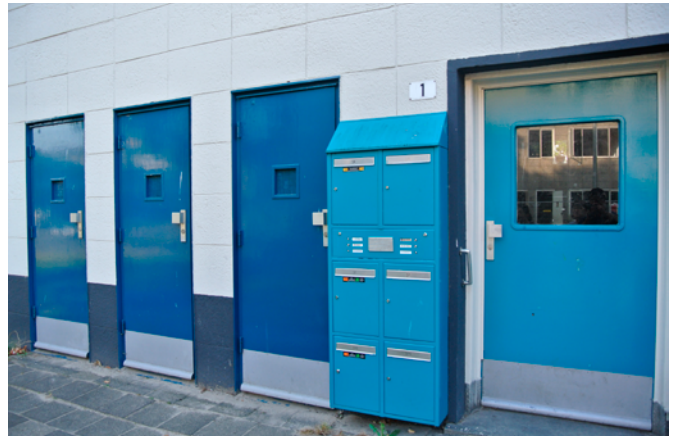
Amount : strip (A) 21 / strip (B) 25 Material : Steel (doors) Size : 1250 x 2250mm (entrance door) 900 x 2250mm (storage door)
