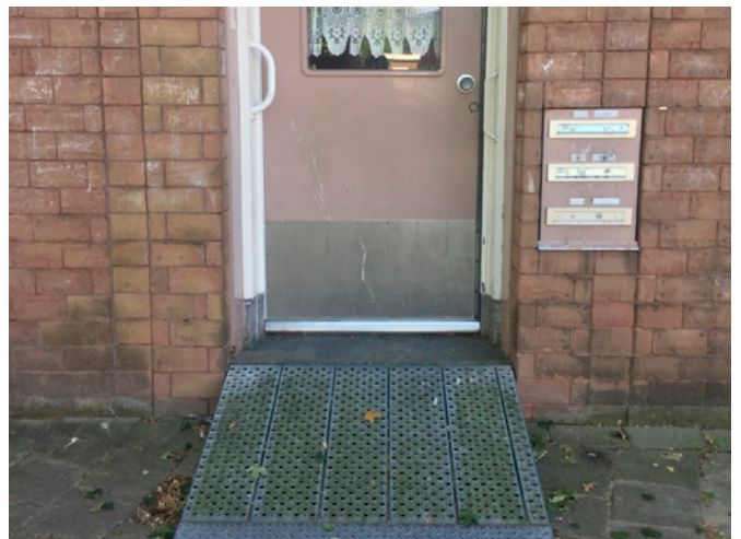
Image 6.10: Slope in front of the door
