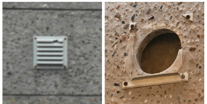
Amount : strip (A) 60 / strip (B) 71 Material : Plastic (ventilation grill) Size : \phi 100mm
