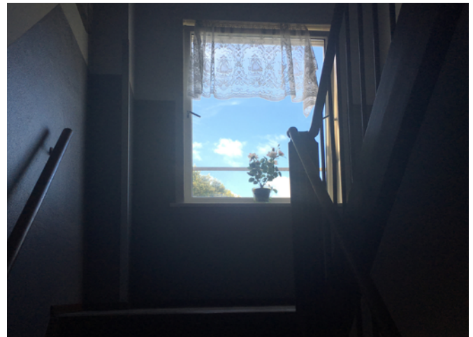
im. 4.5 The window in staircase in Airey block
