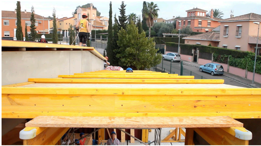
The construction of the roof of the dinning room
