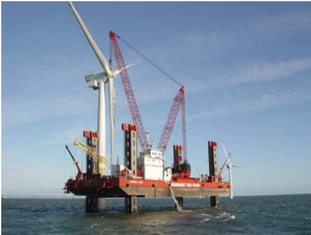
Figure 40. Jack-up barge for heavy subcomponents' repairs
