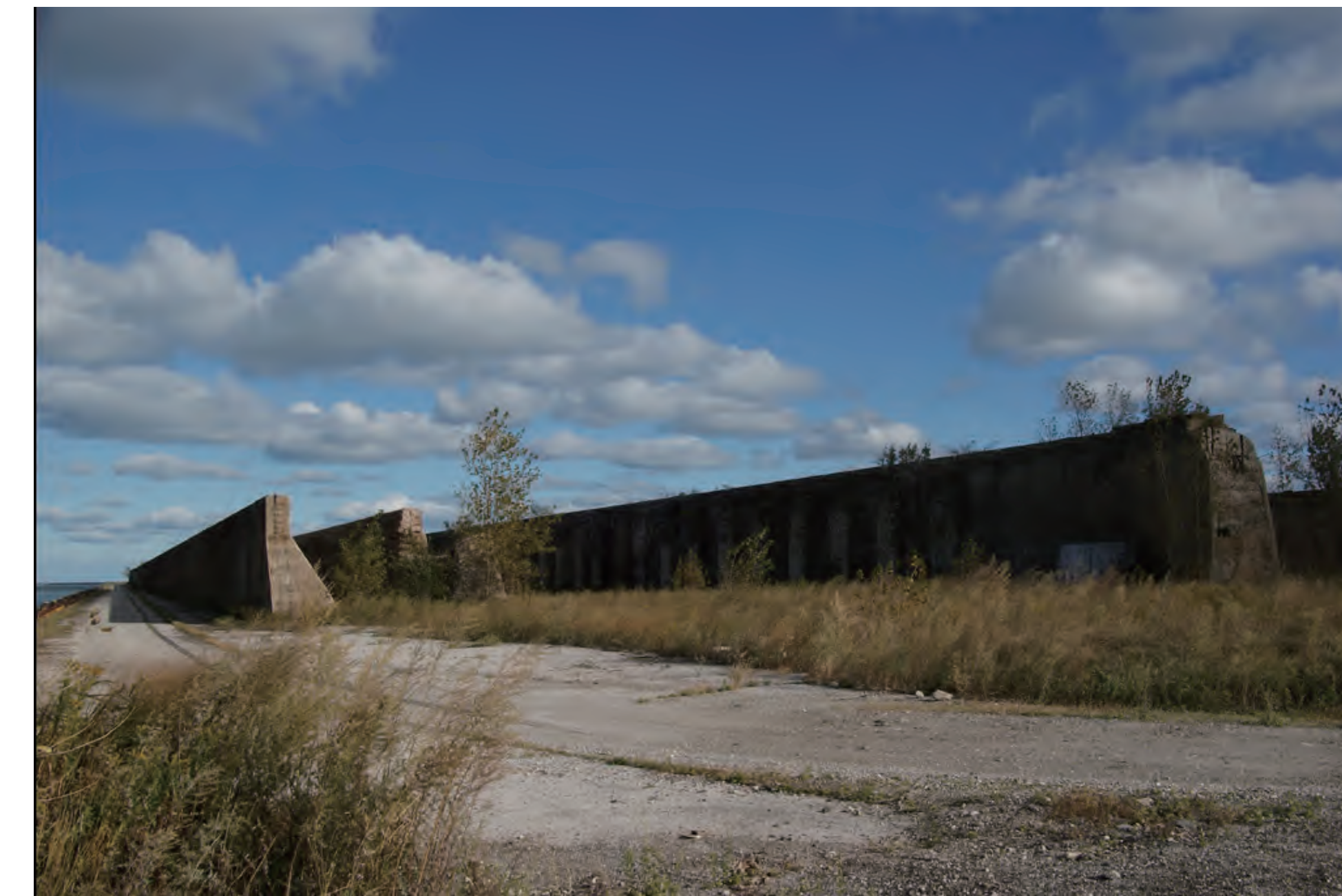
CONDITION OF ORE WALLS
