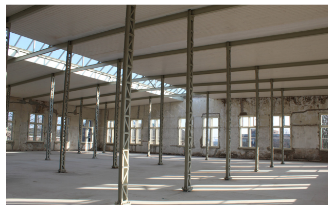
Second Floor Building 8
