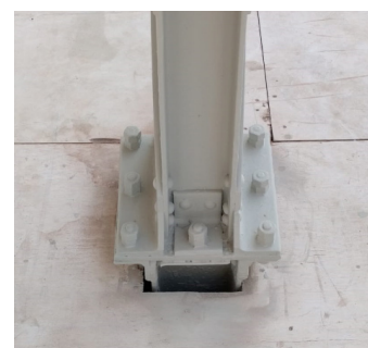
Picture: column through floor
