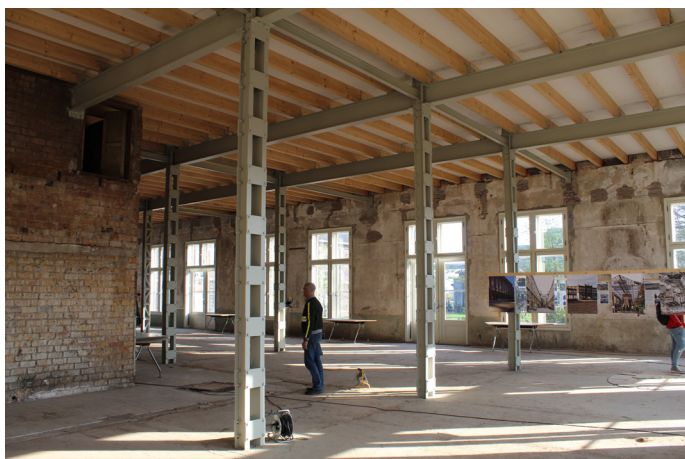
Construction Building 8 source: own image
