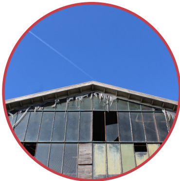
Wired glass façade
