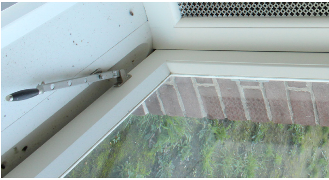
Window Frame Building 8 source: own image
