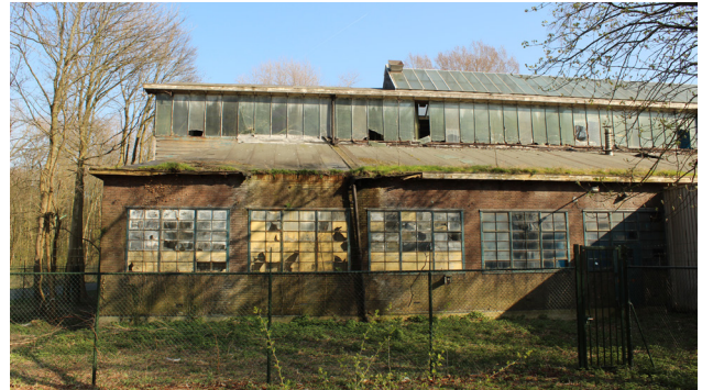
Side Façade Building 320
