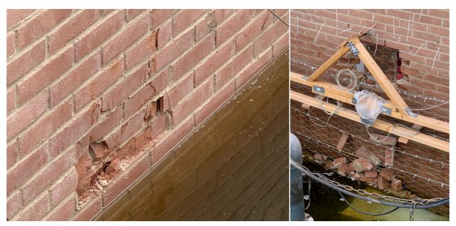
Figure 12. Left, local damage of the bricks led to a hole in the wall, right. The broken and displaced bricks were trapped by the steel net.
