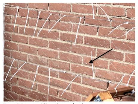
Figure 13. Diagonal stair-like crack pattern from the centre going upwards.
