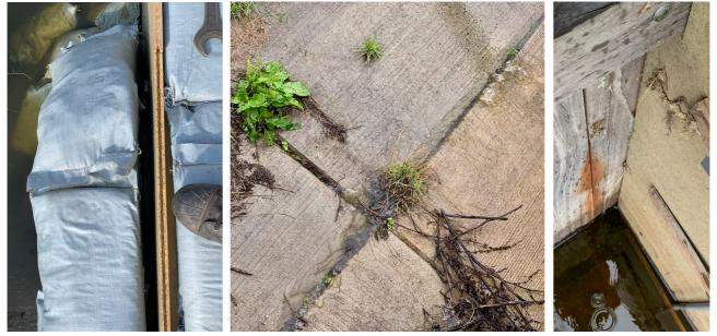
Figure 17. From left to right: gap in the dike, water flowing out of the concrete gaps, and sliding back of the frame.
