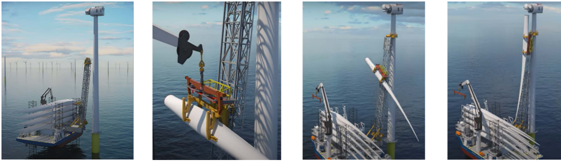
Figure 8.1: Sjøhest Wind Blade Installation Solution by GustoMSC [46].
