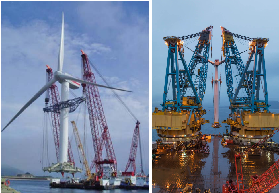
(a) Single lift installation at Beatrice wind farm [20]. (b) Single lift installation at Hywind Scotland [27].
