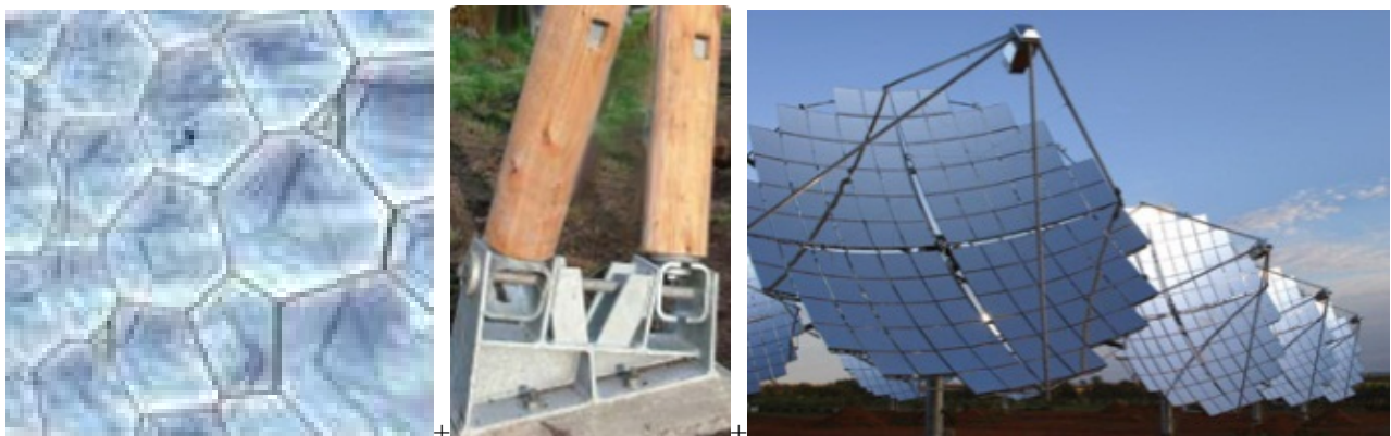
Fig. 3 ETFE cushions + Tentech round wood connection + PV concentration.
