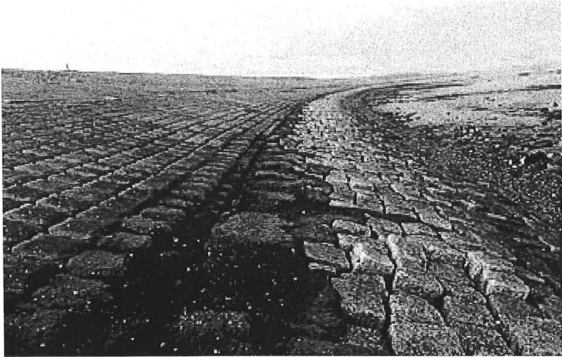
Re-use of granite block on regular granular fill layer
