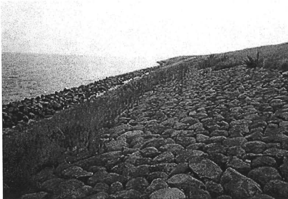
Granite boulders (an old type of pitching, found on the dikes along the IJsselmeer)
