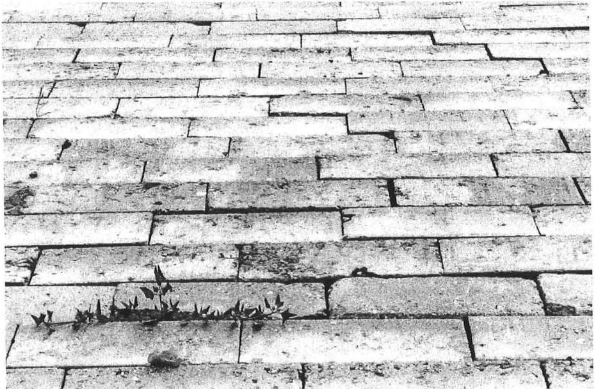
Re-use of concrete blocks, turned on the side
