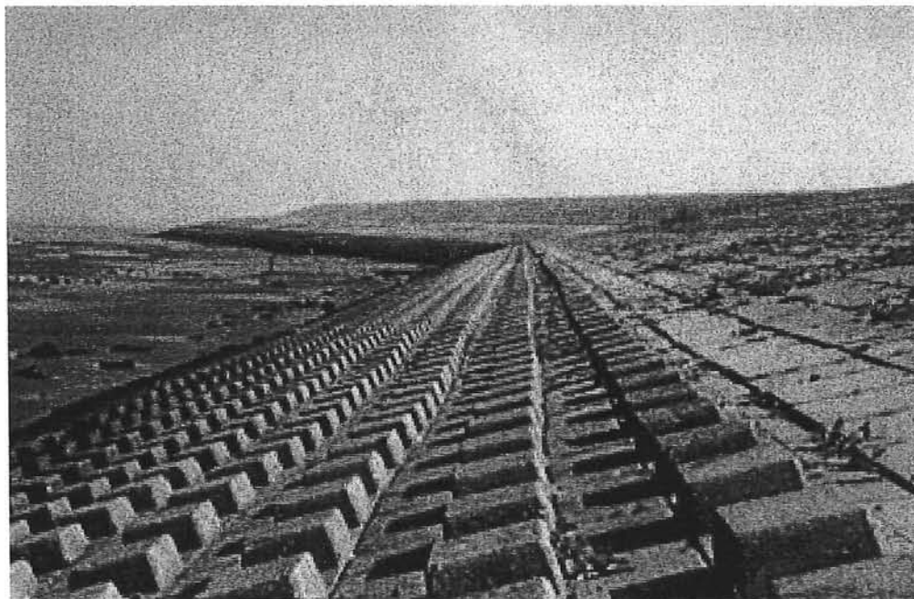
"Diabool" concrete blocks (an old type of pitching, to reduce wave run-up)
