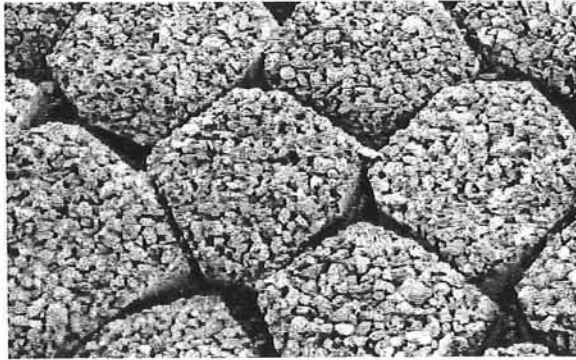
Concrete columns with "eco-top"
