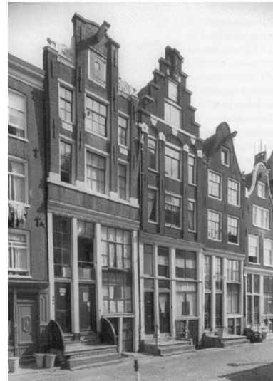
Amsterdam 17th century, Merchant Houses; Bantammerstraat Source: Meischke R. (1995 ); Huizen in Nederland, Amsterdam ; Waanders Publishers Vereniging Hendrick de Keyser / p.48
