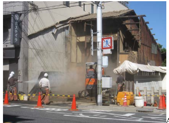
Demolishing a Machiya takes one day! Photo: Alex de Wolf
