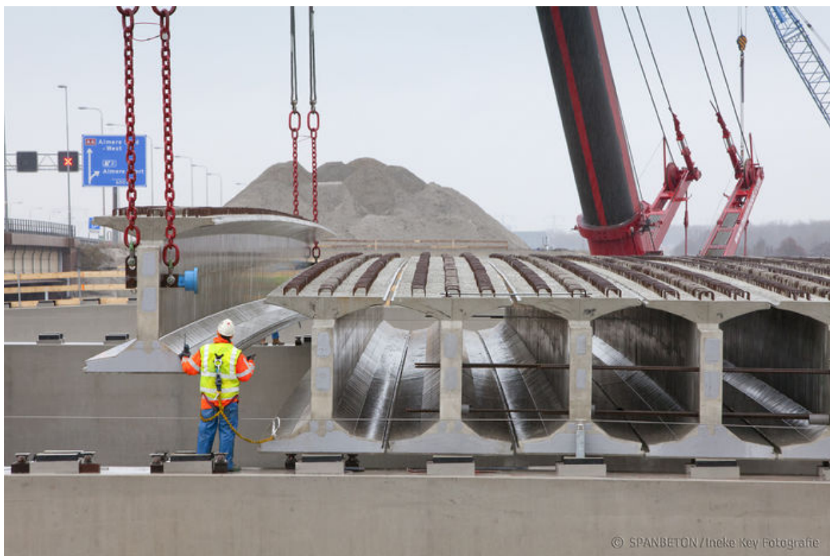
Figure 2.21: Construction of a bridge span with I-beams. Source: Spanbeton
