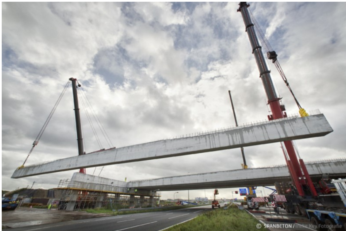
Figure 2.16: Construction of box girders with a span of 61 meters across the Dutch highway A12 near Zoetermeer. Source: Spanbeton, photo by Ineke Key Fotografie
