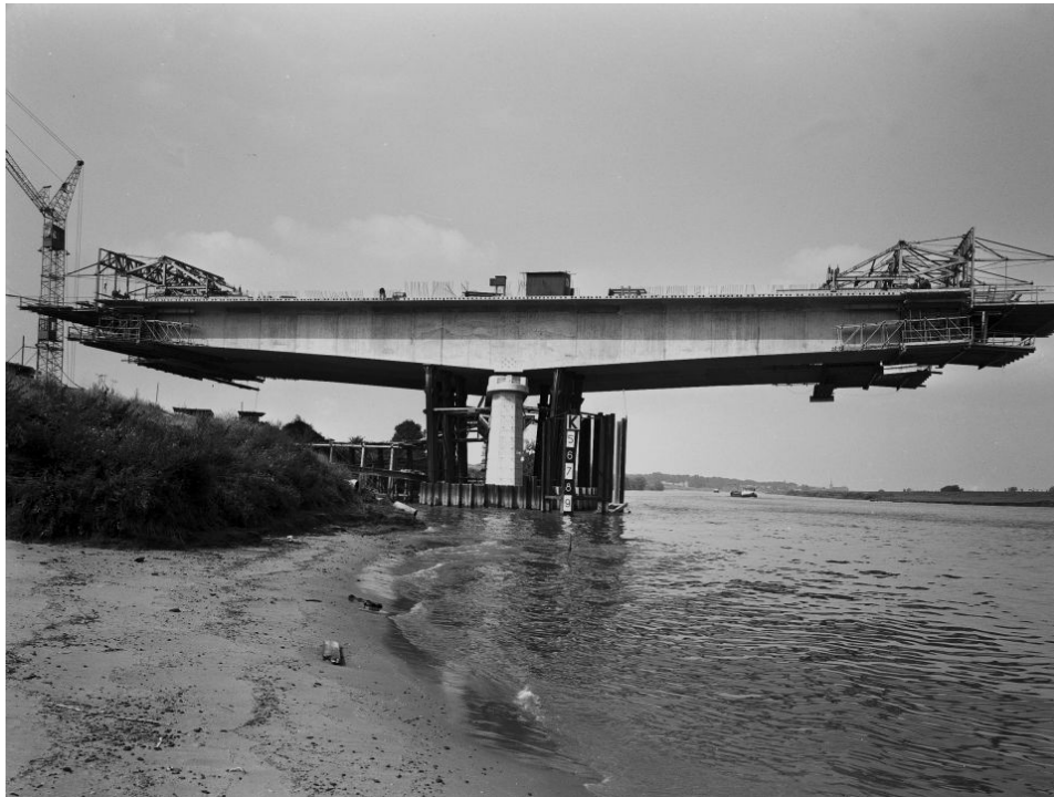
Figure 2.9: Cantilever bridge at the A67 across the river Maas, Grubbenvorst 1967. Source: Cement article: "Maasbrug Grubbenvorst beoordeeld" in number 7 2017 [13]
