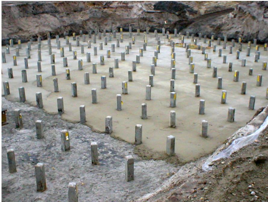
Figure 2.28: Prefab concrete foundation piles in a rectangular grid. Source: De Groot Funderingstechnieken NV, www.dgft.eu/funderingen/fotos/palen/geheide-prefabpalen-2/
