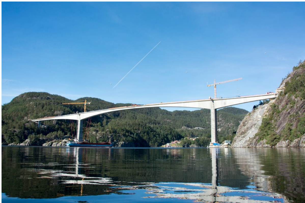
Figure 2.14: Largest balanced cantilever bridge of the world, Stolmabrua in southwest Norway. Source: www.vareveger.no/artikler/rekordbrua-er-ferdig/224727
