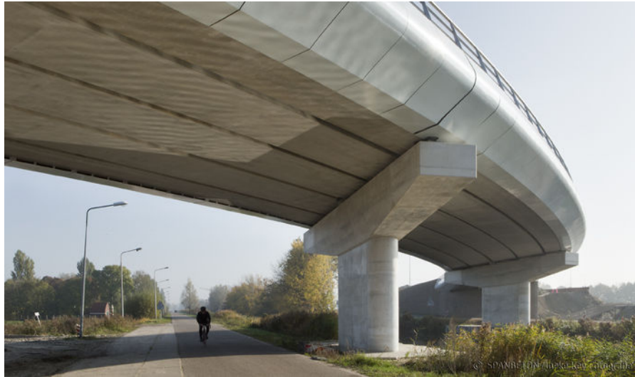
Figure 2.26: Fly-over with box girders supported by capping beams. Source: Spanbeton
