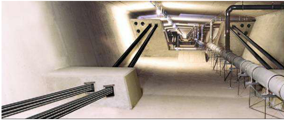
Figure 2.13: External prestressing in a balanced cantilever bridge. Source: Schäfer Bauten, www.researchgate.net/figure/Inside-of-a-box-girder-of-a-post-tensioned-concrete-bridge-with-deviated-external_fig3_242280102
