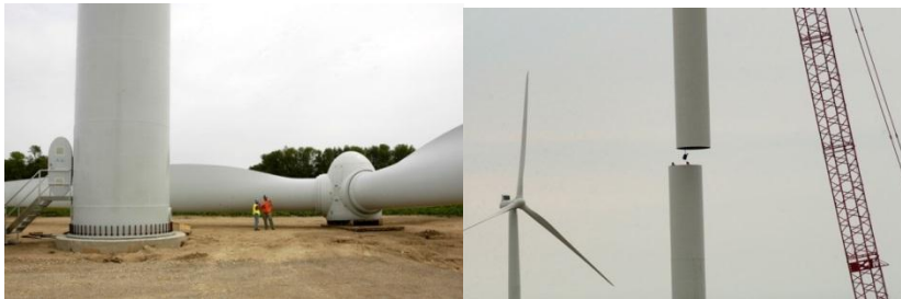
Figure 128 ... (left) Rotor disassembled from tower and (right) disassembly of the tower in parts (Mlife.com, 2008)
