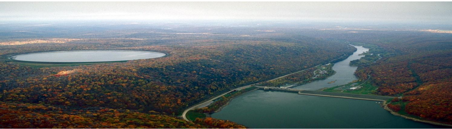
Figure 34 ... Seneca Pumped Hydro Storage Plant near Pennsylvania, USA (Wikipedia, 2010)
