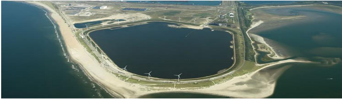
Figure 63 ... Aerial view of the Slufter (Portofrotterdam.com, 2013)
