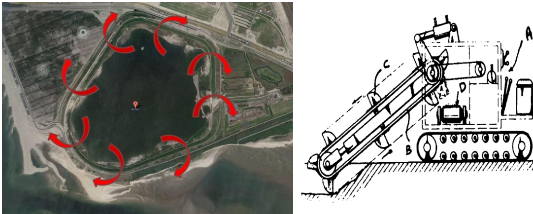
Figure 139 ... (left) Pumping of the silty clay material from the inside to the outside of the dam and (right) Example of bucket wheel excavator (USPTO.gov, 2013)
