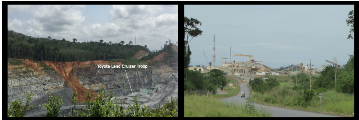
Figure 2-1: Picture of Main Pit with Focus on Northern Footwall and Processing Facility Left: Main pit with major slope failure. Toyota Land Cruiser (white 'dot') for scale indication. Right: processing plant with primary stockpile on right side with feed from gyrotary crusher.
