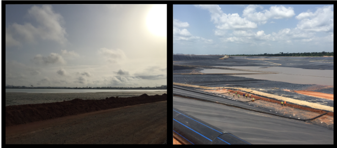
Figure 2-8: Picture of Tailing Storage Facility Cells
