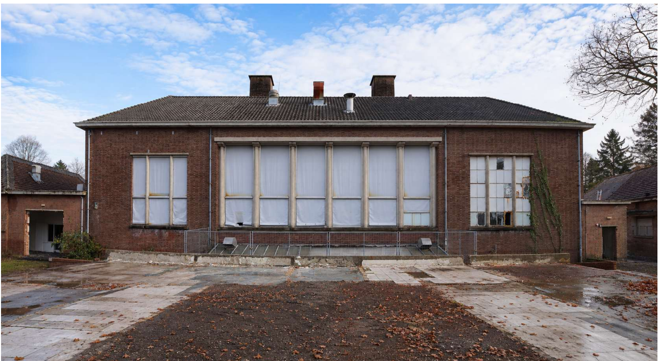
Figure 312 - top: Building 13's east facade (author's work)
