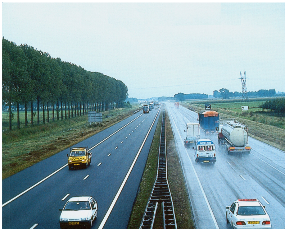
Figure 2.12. – Effect of rain on Open Asphalt Concrete (left) and Closed Asphalt Concrete (right)
