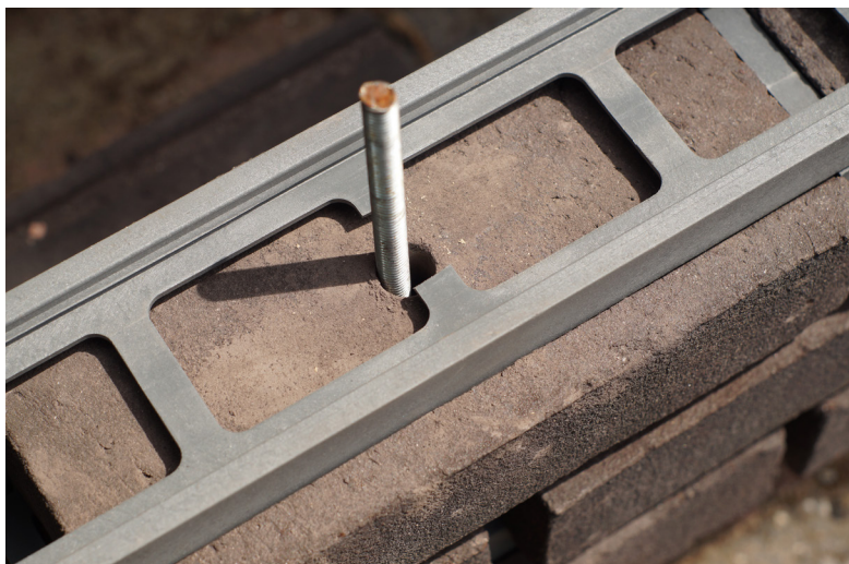
figure 117, Profile adapted for tension rod
