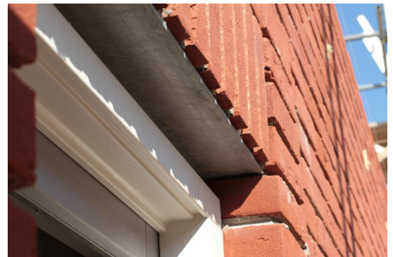
figure 19, Steel lintel in use
