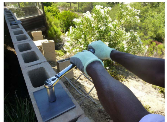
figure 115, Tensioning by hand
