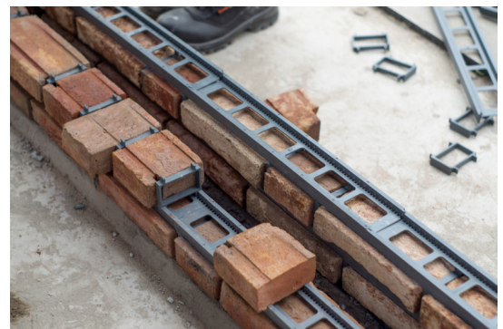
figure 07, H-block during construction at The Green Village
