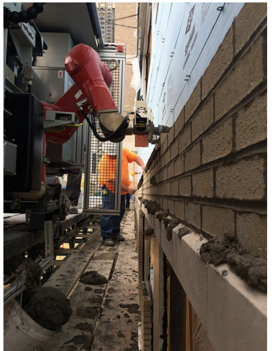
figure 04: Construction worker working next to SAM100 robot.
