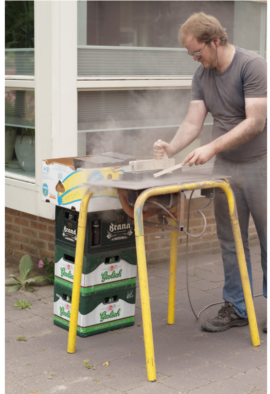
figure 119, cutting the channels
