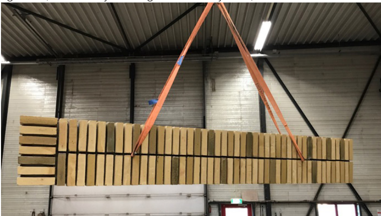
figure 21, Verbaan systems' glued masonry lintel,
