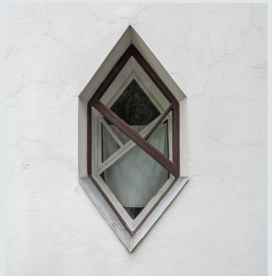
figure 72: Finished window at Melnikov house
