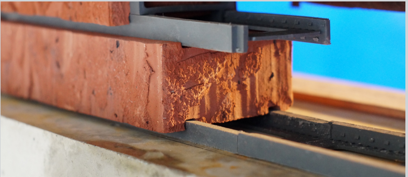
figure 26, Half H-profile on concrete
