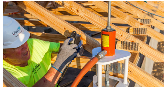
figure 113, Tensioning with pneumatic tensioning bridge
