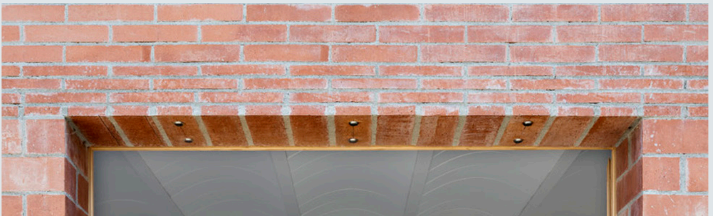
figure 99: Lintel construction of Casa 1219
