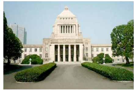
National Diet Building, 1936, arch: Ministry of Finance Architecture Department
