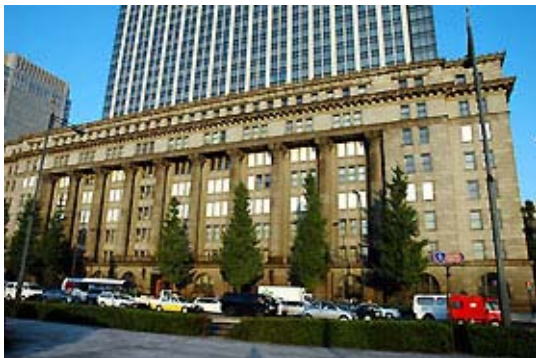
Tokyo Marunouchi, Meiji Life Insurance Building, 1934 architect: Shinichiro Okada, bouw Takenaka Corporation
