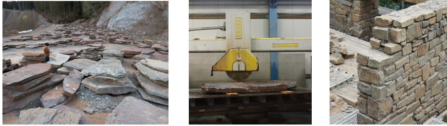
Figure 4. Collecting, sawing and stacking stone for Woodstock by BC Architects
