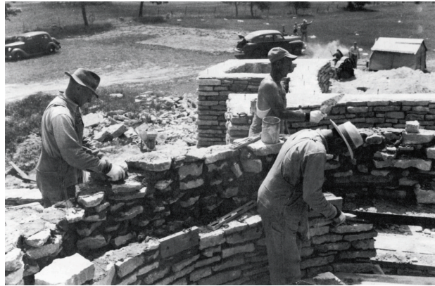
Figure 2. The Jacobs House 2 by Frank Lloyd Wright, under construction
