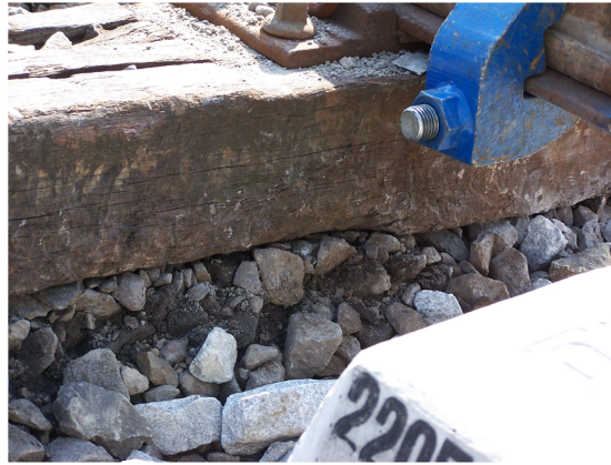
Fig. 1. Severely wore ballast stones under an old sleeper. Compared with the new ballast stones nearby with sharp edges, the wore ballast stones have become rounded in shape and covered by dusts. This problem is called the “foul” of the ballast, meaning that the ballast stones have been crushed, provide less drainage, move less and have less elasticity, leading to a reduction in their friction dissipation.
