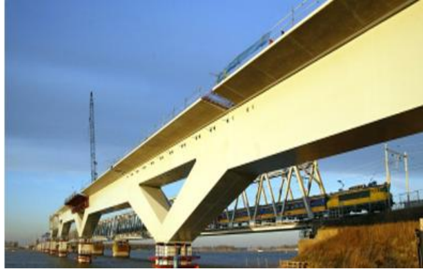
Figure 56. Typical steel bridge
