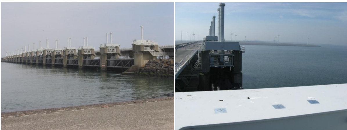
Figure 22. Left: Overview of a section of the Oosterscheldekering Right: Close-up of a single sluice.
