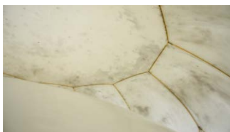
Figure 18: Removal of the inflatable mould
