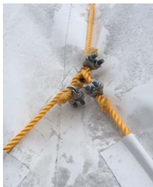
Figure 14: The joint connection of the cables
