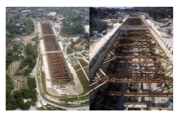
Figure 1-1: A typical cut-and-cover excavation of a rectangular shaft. Notice the web of struts required to keep the shaft in place. Photo: oasys-software.com
