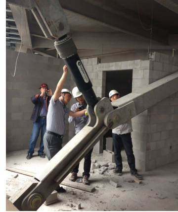
(b) Viscous damper in practice
