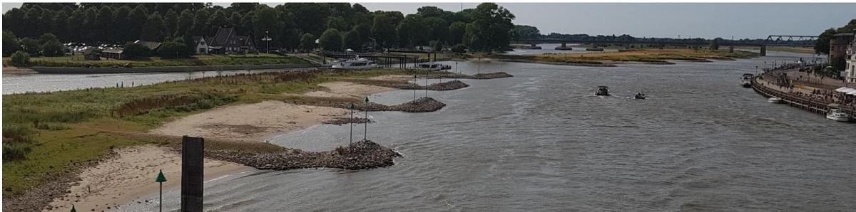
Figure 1.2: Innovative island groynes in the River IJssel at Deventer during extreme low water levels in July of 2018. In the background, under the railway bridge and at the left the excavated floodplains, constructed for Room for the River, are visible (Photo: Lindert Ambagts)
