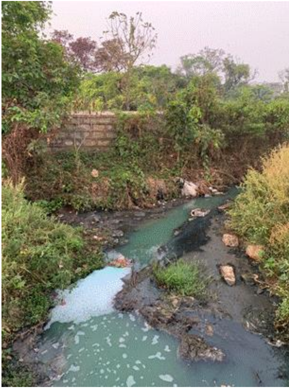
Figure 14: Stormwater drain from SMV layout meeting the main inlet drain (left) Overflowing last manhole in the lake catchment where grab sample was taken (right)
