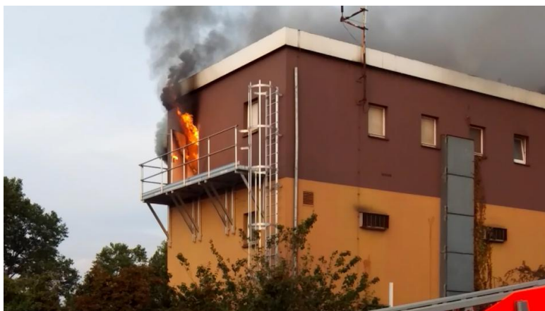
Figure 4.17 Fire in the relay room inside a signal box in Mülheim (WDR, 2016)
