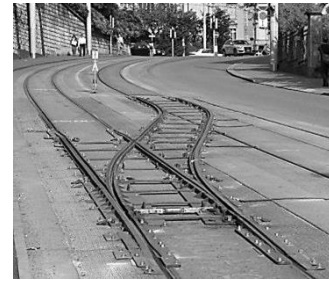
Figure 2.4 Sketch of how to assemble a Californian switch (left) and a Californian switch in use (right)
