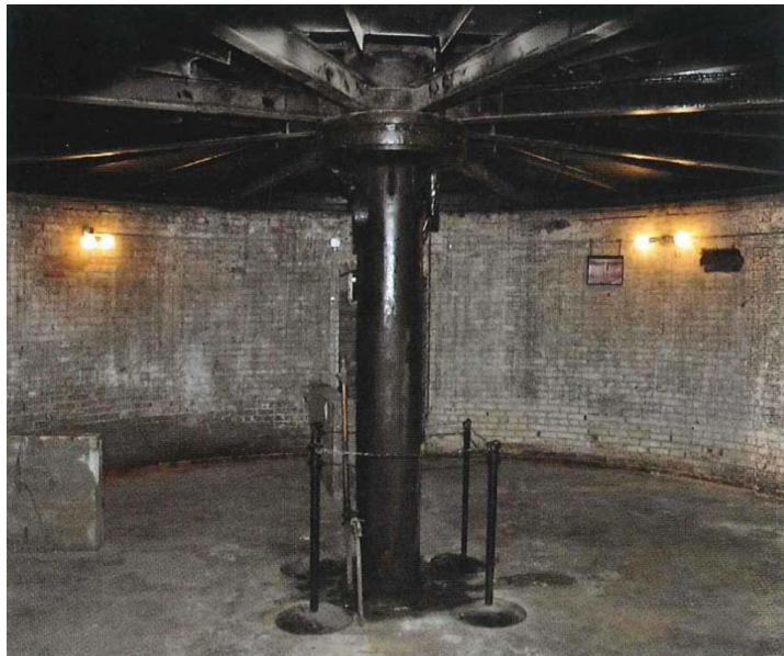
Figure 28: Rotating mechanism of a rotating jail
