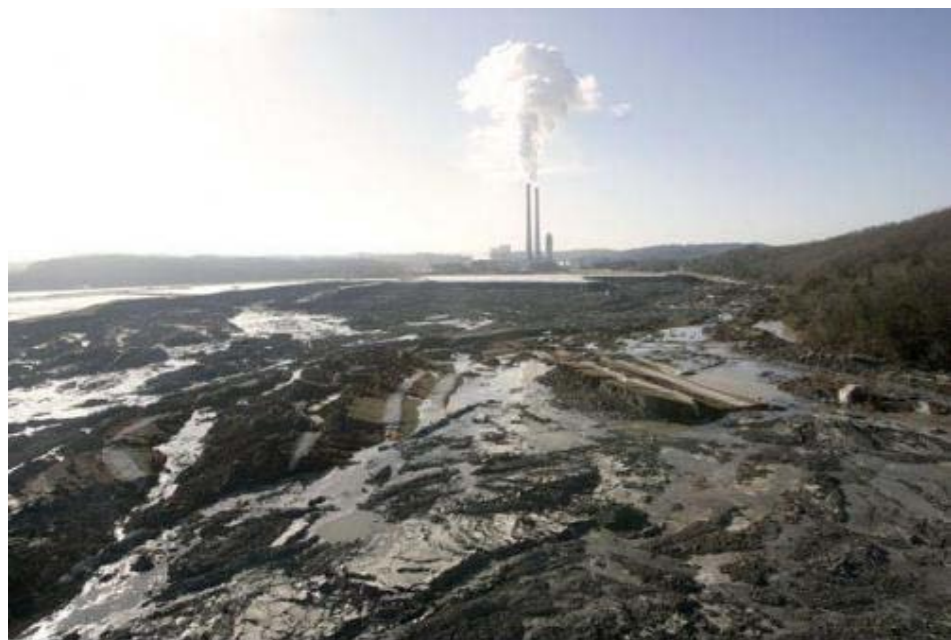
Aftermath of a retention-pond-wall collapse
