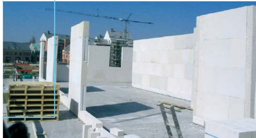
Fig 99: Partially built walls 24
