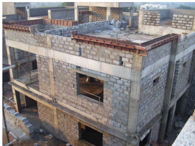
Fig 4-8: A typical example of conventional construction of housing, in Bangalore
