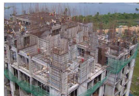
fig. 26,27- mivan formwork system- RC box frame construction
