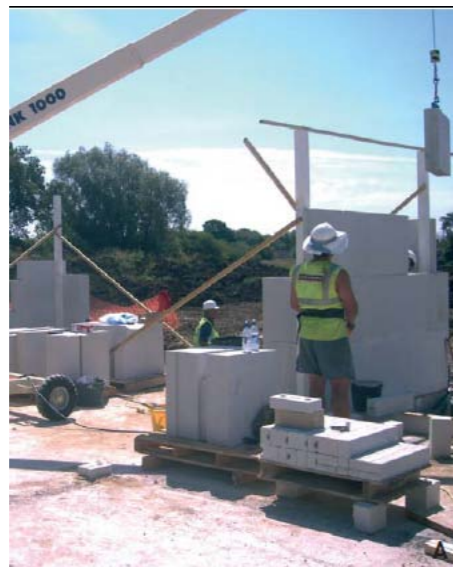
Fig 97: mechanical lifting and placing of a panel 24
