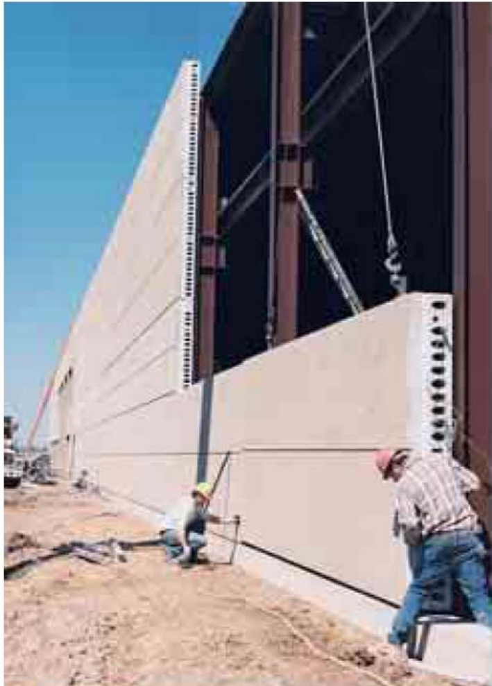
Fig 84: An industrial building with sandwich panels 21
