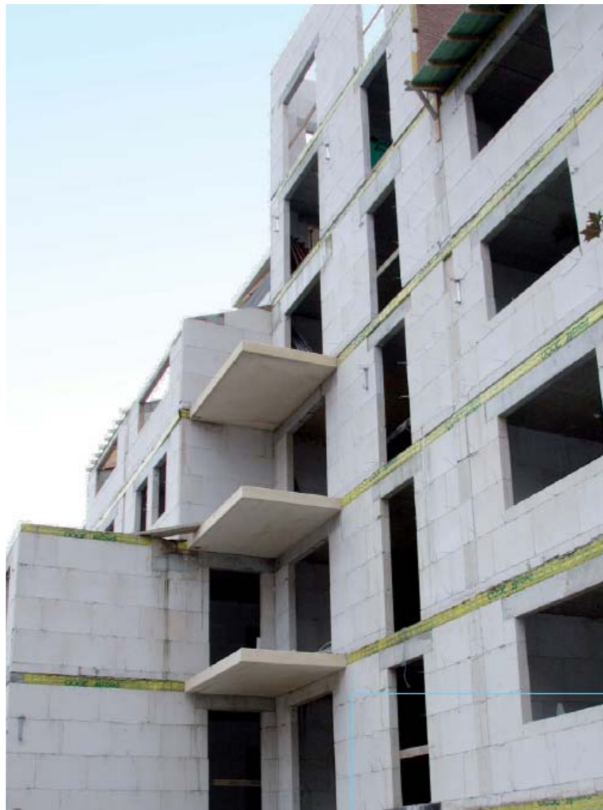
Fig 102: view of unfinished SILKA wall 24
