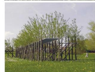
Figure 2.2 on the bottom shows *Der Steg*, a walkable canopy with columns made of living willows, constructed in 2005. First, several willows were bonded together to ensure its initial strength. Over time the willows grew together into interconnected elements.
