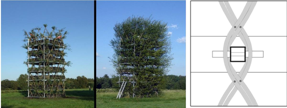
Figure 2.3 Left: Baubotanik-Tower after completion, Middle: and one year later (Ludwig, 2014). Right: Willows around a connection (Ludwig, 2012)
