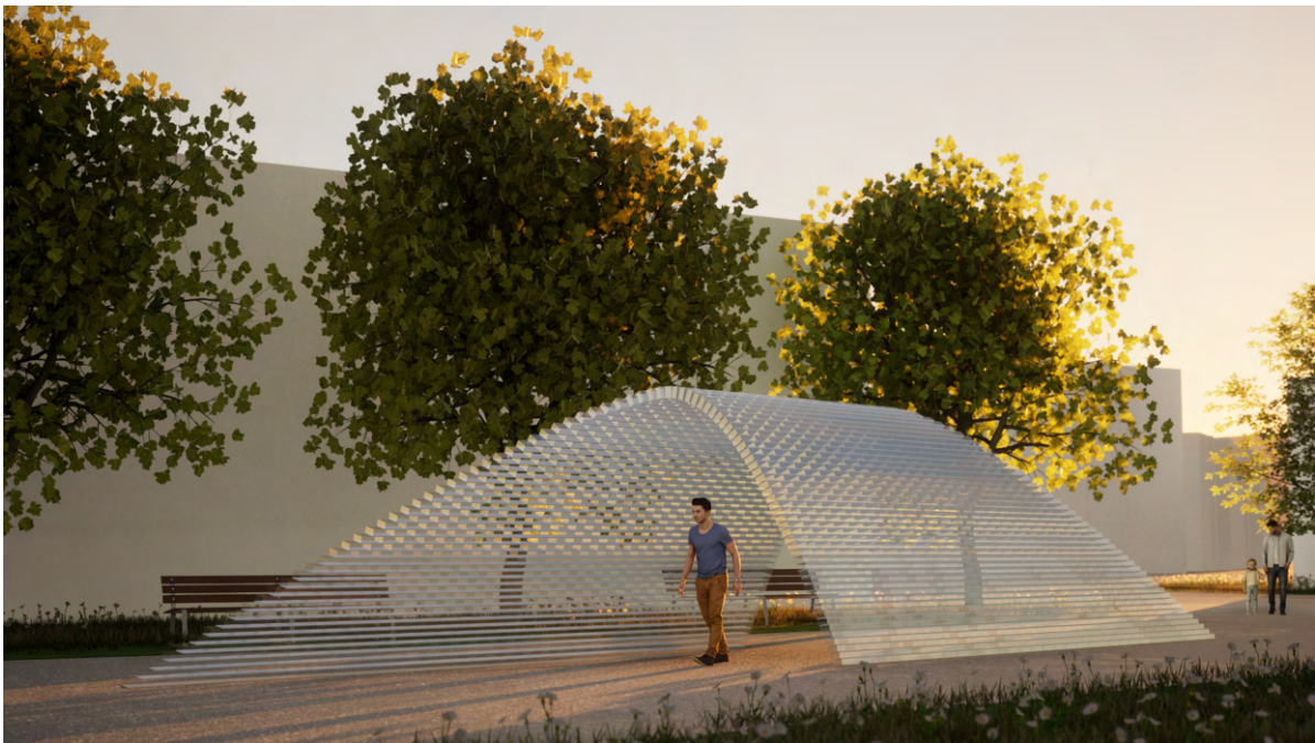
Figure 7.10: Render impression of the demountable glass vault, illustrating the overall geometry and transparency of the structure
