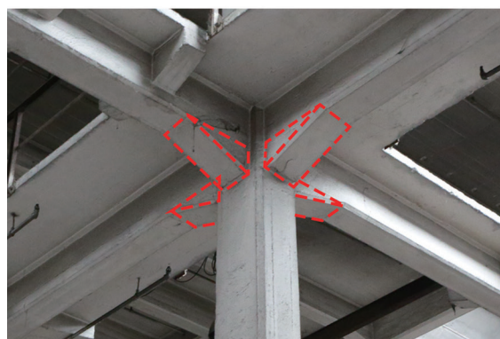
brackets of the beams
