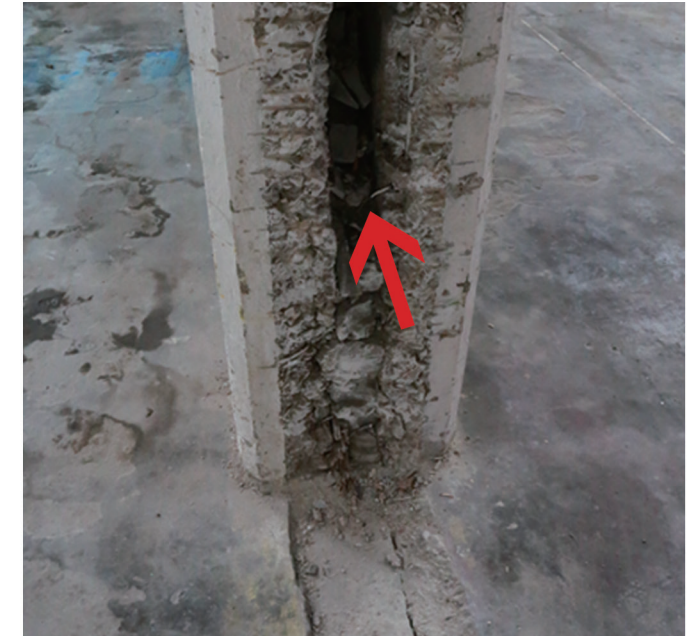
The cavity between compartment walls
