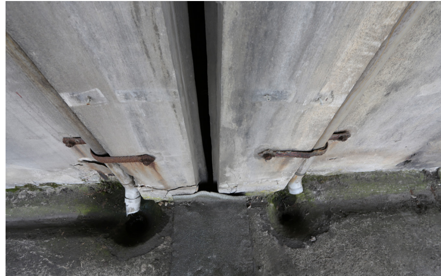
Two symmetrical drainage pipes and holes on the both sides of the compartment walls.
