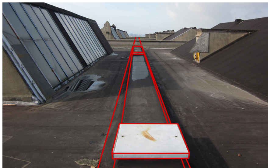
fig1.The tube in the middle of the roof that contains electrical wires for the building.
