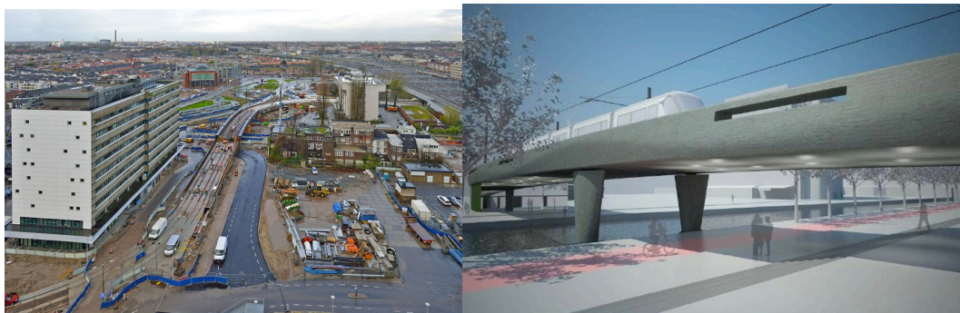
Figure 10 HOV-viaduct under construction (left) and the design (right) (Boekel, 2016)
