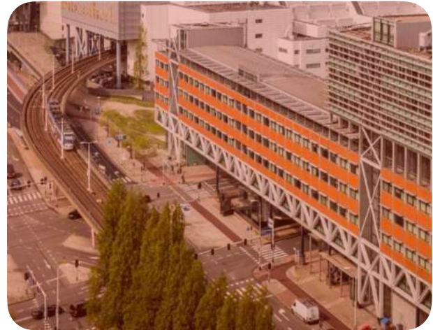
Figure 8. The Hague Tech building (CID, 2019)
