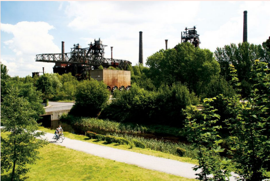
Figure 147: Dispersed collection of former industrial structures (Groenblauwe Netwerken, n.d.).
