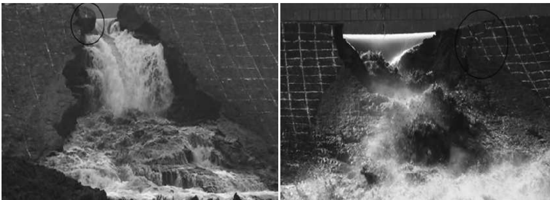
Figure (2 - 2): Damping failure (left) and shear failure (right) (Zhang et al. , 2009)
