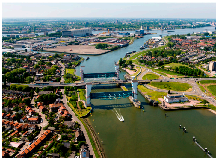
Figure 5. The Hollandse IJssel storm surge barrier as it protects the Hollandse IJssel located behind it. Courtesy Rijkswaterstaat, mediatheek.
