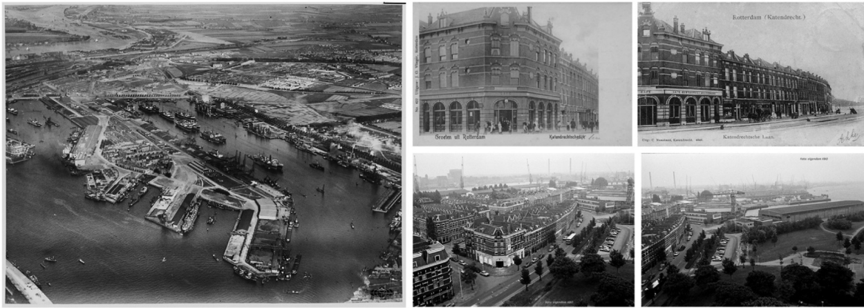
Figure 1. Left: aerial image of katendrecht, 1922 (municipality of Rotterdam, city archives). Right (two above): 1900 – café restaurant belvédère (municipality of Rotterdam, city archives). Right (two below): 1981 – the belvédère, Katendrechtse Bewonersorganisatie (KBO).
