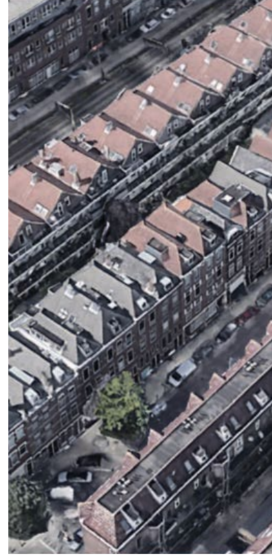
Row house; Rotterdam
