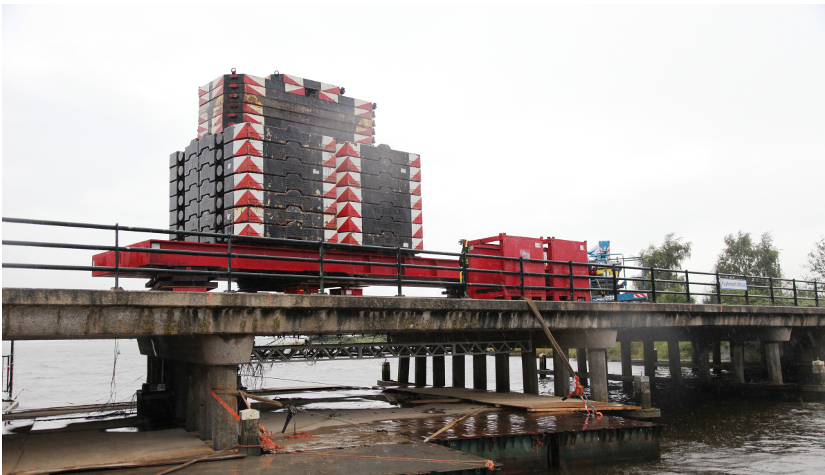
Figure 1.1: Proof loading on a bridge executed by Lantsoght et al. [16].
