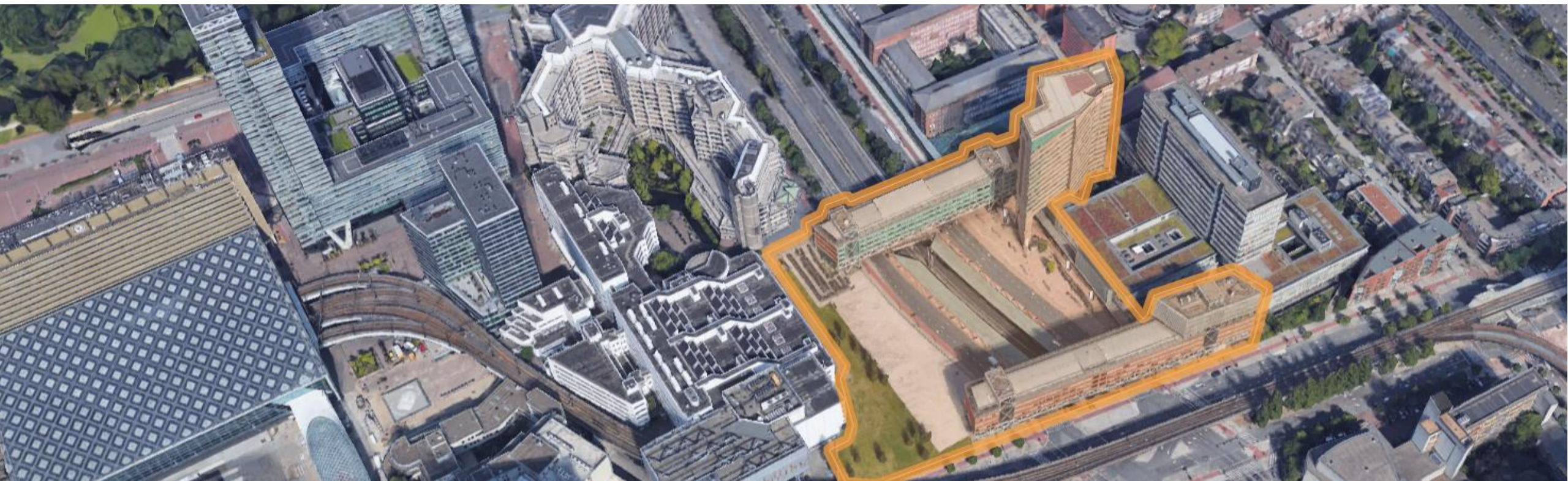
BRUGGEBOUW-EAST Build in 1999 as part of a cluster of buildings Part of the Government in 2017
