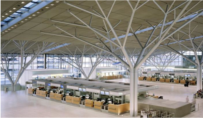
Figure 106: Tree shaped columns at airport Stuttgart.
