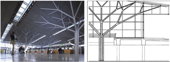
Figure 107: Schematization of tree shaped column.
