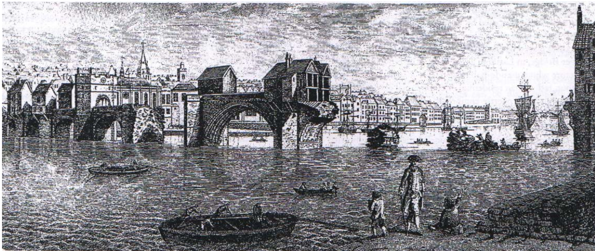
Figure 3.3: Old Tyne Bridge, Newcastle, in ruinous state, 1772.
