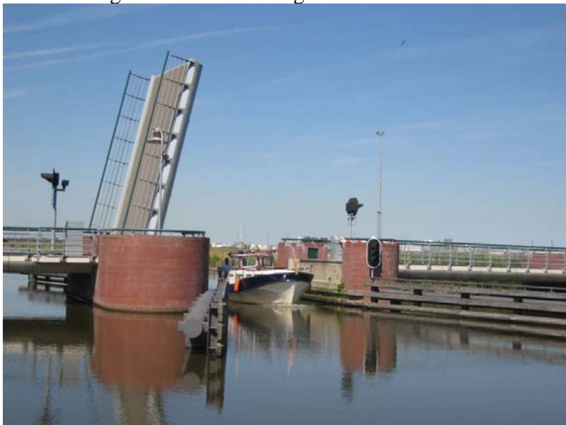
Figure 8.16: Movable bridge with a contra-weight
