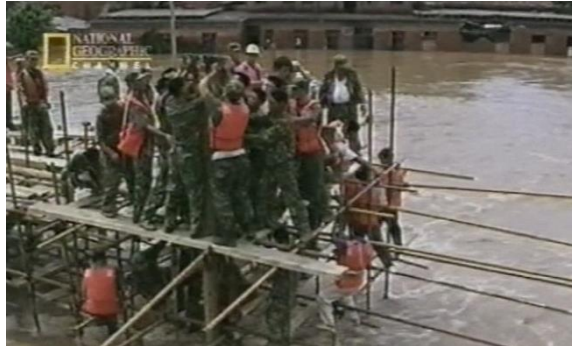
Figure 3.20: Construction of a scaffold, (Rage of the River Gods, 2001)
