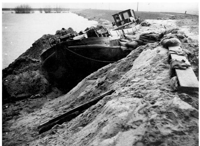
Figure 4.7: Ship the 'Twee Gebroeders' after emergency closure, source: Nationaal Archief/Spaarnestad Photo/ANP ©
