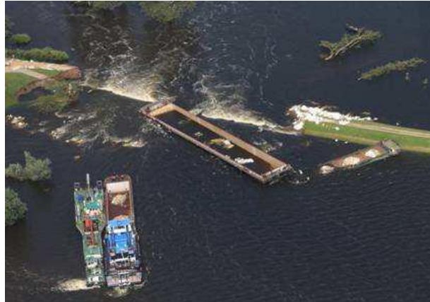
Figure 4.40: Barges in the breach as emergency measure, source: dpa photo
