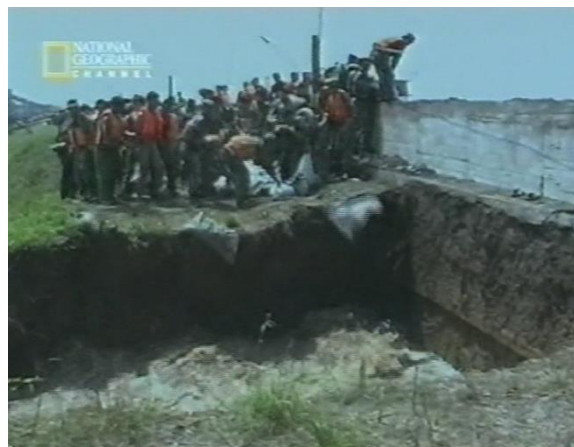
Figure 4.16: Development of the breach under the flood wall (Rage of the River Gods, 2001)
