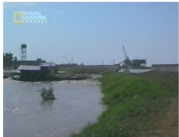
Figure 4.19: Failed emergency closure by means of a vessel (Rage of the River Gods, 2001)
