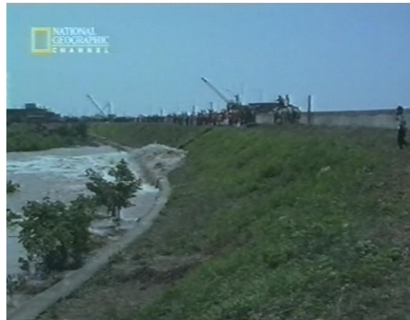
Figure 4.15: Early stage of piping at the City Defence Dike (Rage of the River Gods, 2001)
