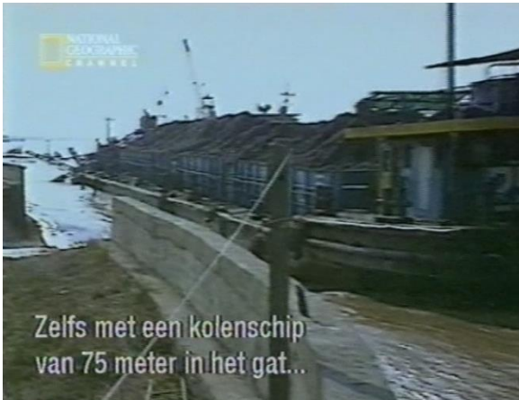
Figure 4.20: Sinking down a freighter filled with coal (Rage of the River Gods, 2001)
