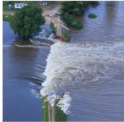
Figure 4.36: Dike breach in Fischbeck, source: AP
