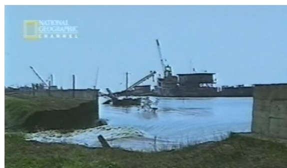
Figure 4.17: Collapse of the City Defence Dike (Rage of the River Gods, 2001)
