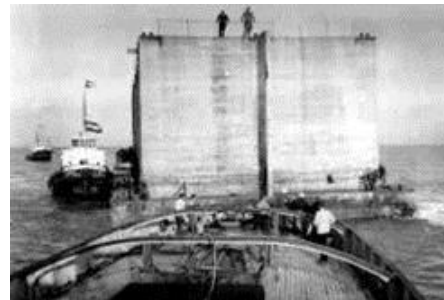
Figure 3.18: Example of a caisson
