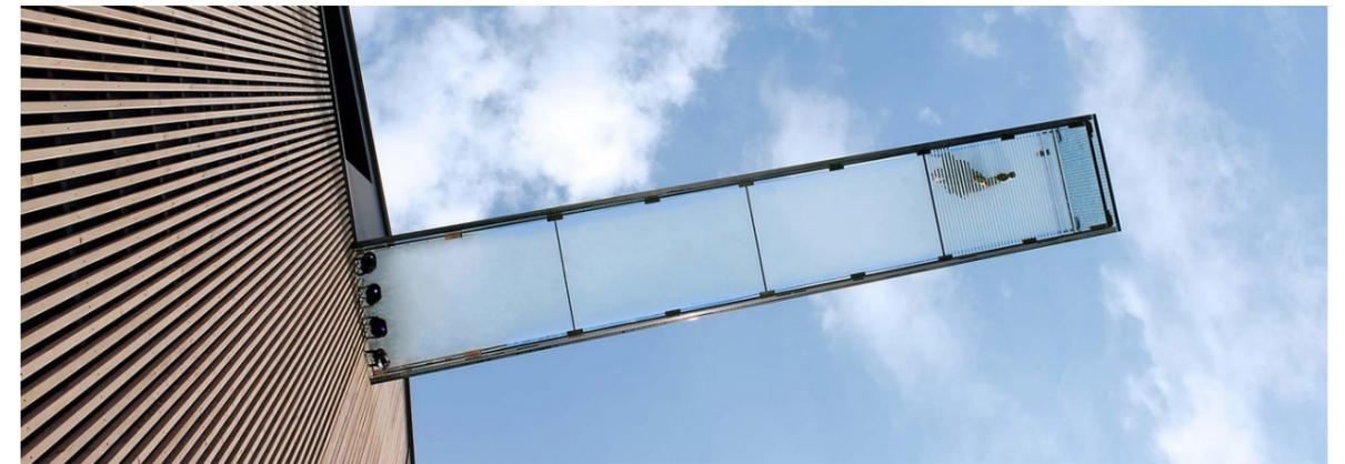
Figure 2 : Bründl Kaprun flagship store sky walk made from laminated float glass (seele, 2021).
