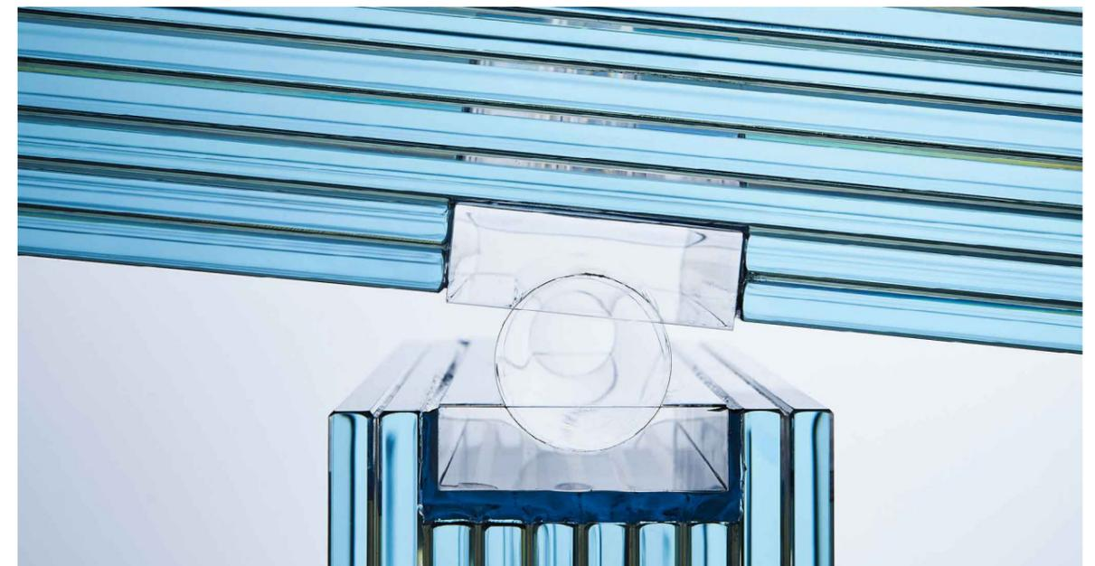
Figure 20 : In the project Glass wipe by (Eckersley O'Callaghan, 2018) were up to 11 layers of glass are laminated using SentryGlass interlayer.
