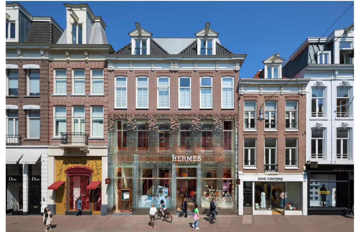
Figure 49 : Transparency of cast glass as seen in the facade of Crystal House (MVRDV, 2016)
