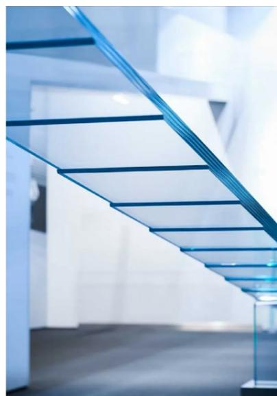
Figure 74 : Directional transparency of laminated glass as displayed in the project Glass wipe by (Eckersley O'Callaghan, 2018)
