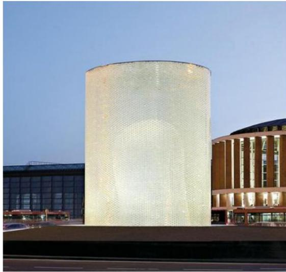
Figure 25 : Atocha memorial, cast glass bricks, image source: (Tensinet, n.d.)
