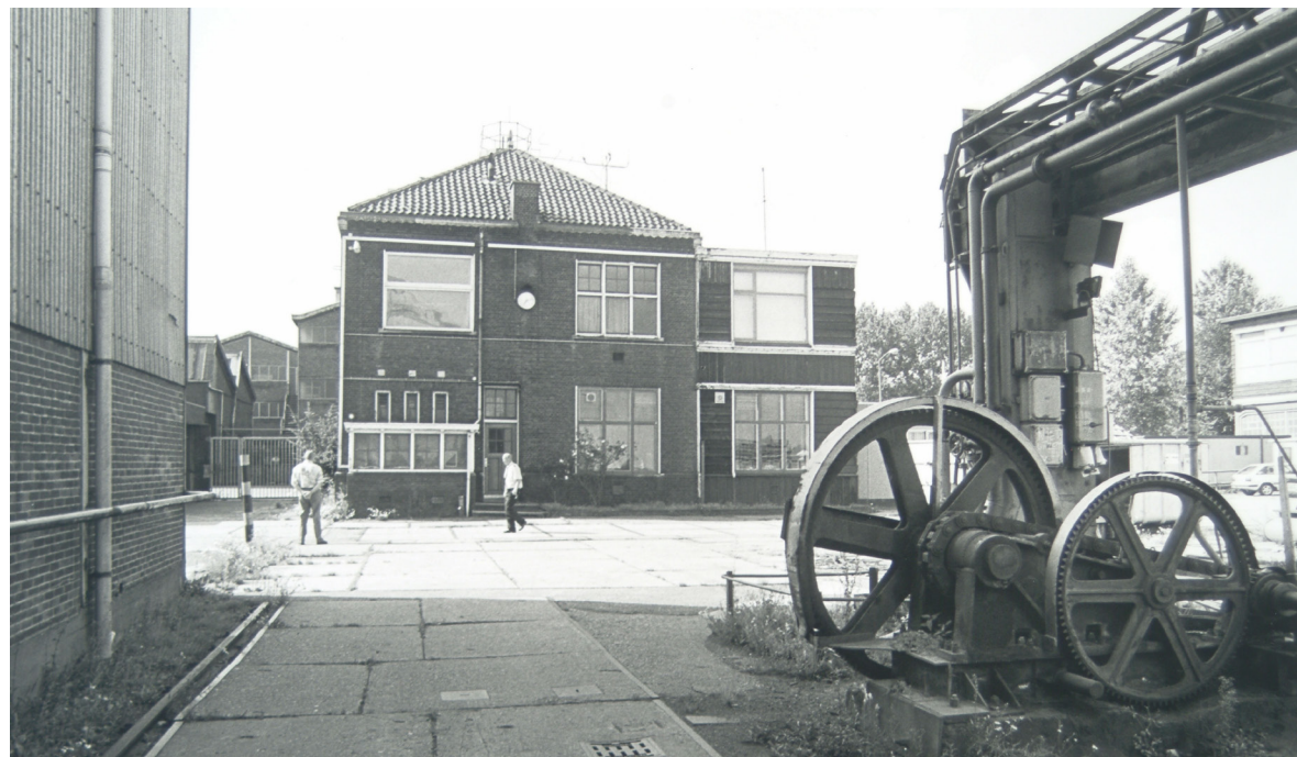
CHARACTERISTIC VIEW INBETWEEN PRODUCTION HALLS, BIESBOSCHHAL INBETWEEN BUILDINGS IN THE BACK, 2000 (Regionaal Archief Dordrecht)
