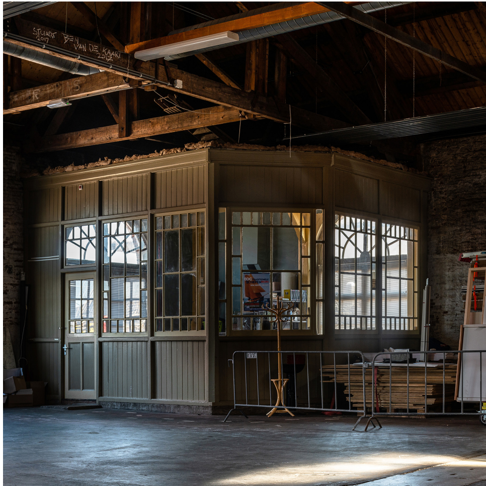
former supervisor's house (winhov.nl)
