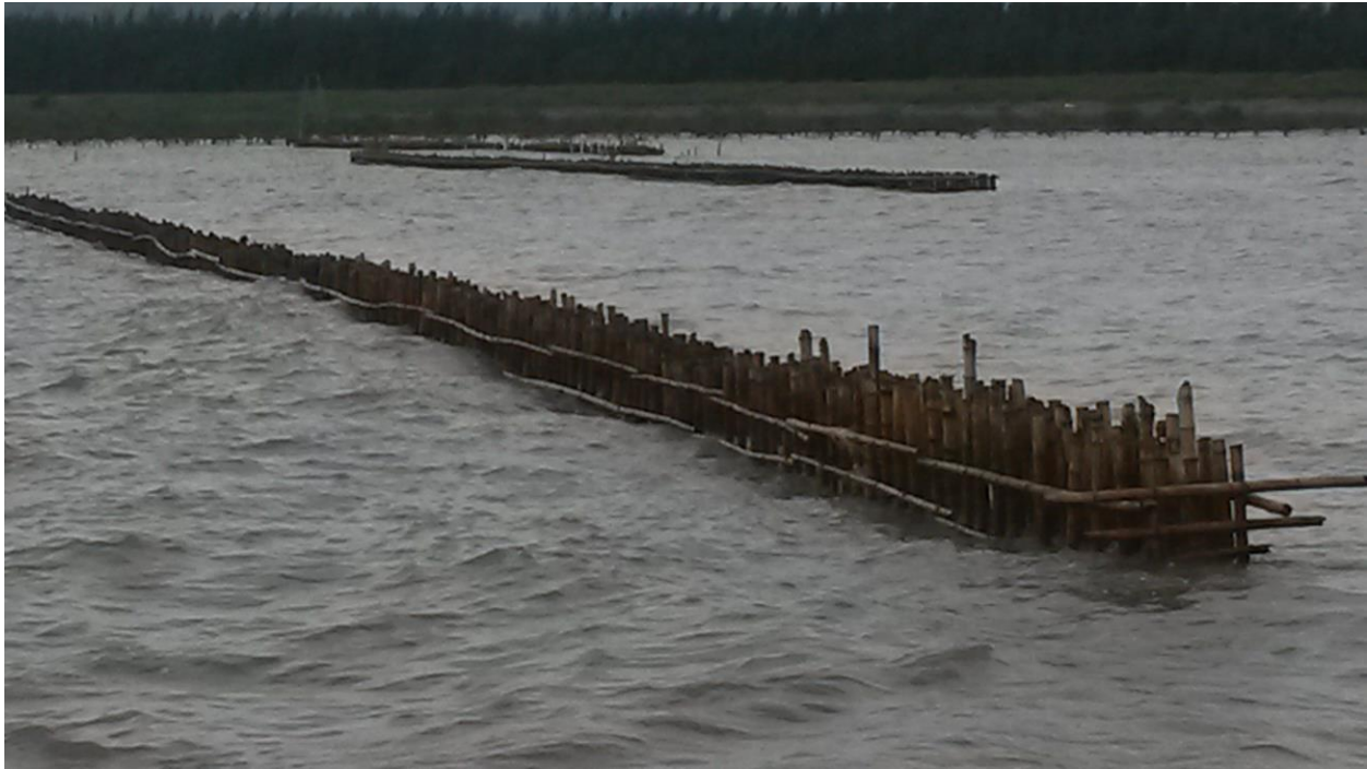
Figure 5-3 Bamboos with reed filling in the gaps being used as wave screens along a T-groyne in Vietnam (picture by H.J. Verhagen)
