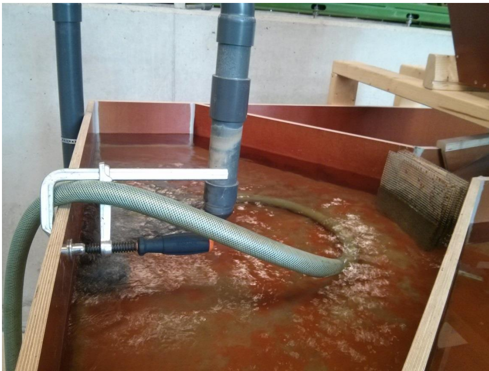
Figure H.16 – Area where the water flows into the flume and fluctuations in the water level are damped.
