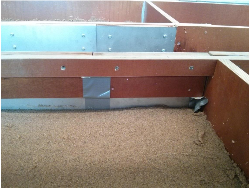
Figure H.5 – Removable bank protections in position with duct tape over the seams to prevent water and sediment flowing through the gap.
