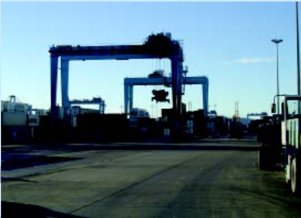
Figure 3: ECO-RTG prototype test site Maersk España terminal in Algeciras, Spain.
