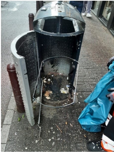
Figure 10 Trash bin with broken internal mechanism
